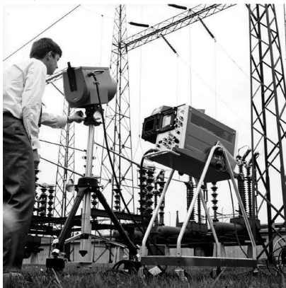
Figure 3.3 LEFT: FLIR Systems Thermovision® Model 661. The photo is taken on May 30th, 1969 at the distribution plant near Beckomberga, in Stockholm, Sweden. The camera weighed approx. 25 kg (55 lb), the oscilloscope 20 kg (44 lb), the tripod 15 kg (33 lb). The operator also needed a 220 VAC generator set, and a 10 L (2.6 US gallon) jar with liquid nitrogen. To the left of the oscilloscope the Polaroid attachment (6 kg/13 lb) can be seen. RIGHT: FLIR Systems ThermoCAM Model E2 from 2002 – weight: 0.7 kg (1.54 lb), including battery.
